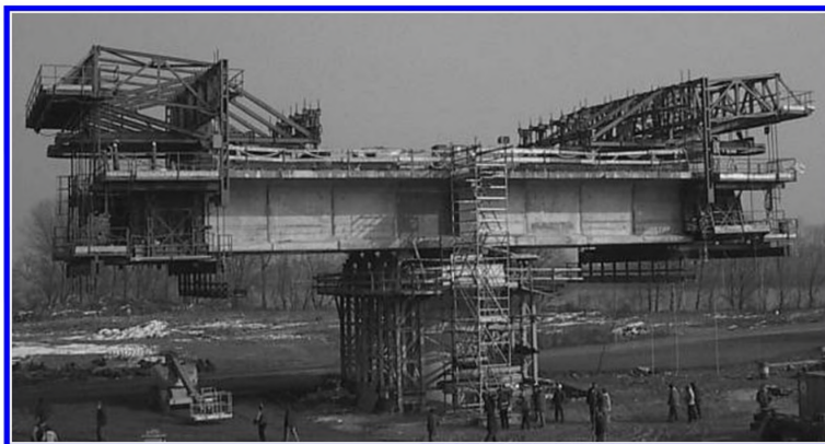
Figure 29. First balanced cantilever of Left Embankment viaduct, approaching cable-stayed bridge over Po River, Milano-Bologna line.
