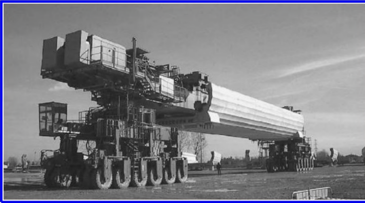
Figure 24. Modena precast deck lifted and transported on tyres from stocking area, Milano-Bologna line.
