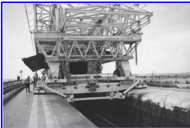
Figure 22. Reinforcement cage transported in the formwork over the piers, Padulicella viaduct, Roma-Napoli.
