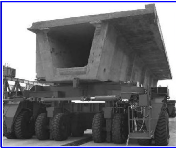
Figure 4. Box girder (type a) on carriers towards launching operations, Milano – Bologna line.
