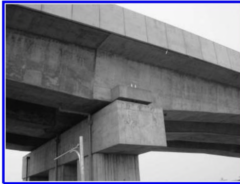
Figure 4. The hold down device located next to the bearings prevents the overturning of the deck.
