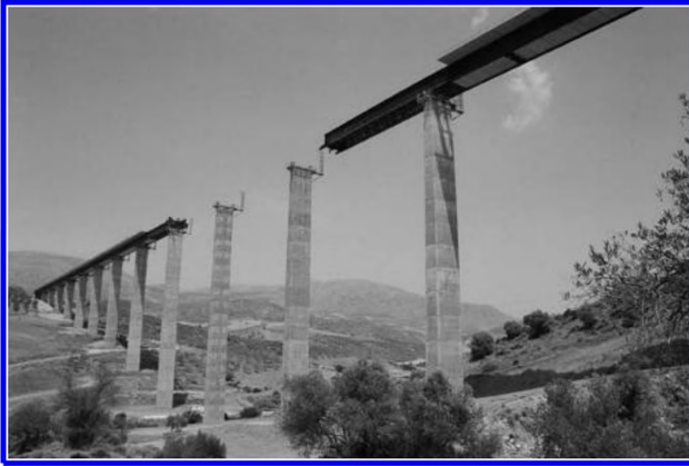
Figure 26. Bridge during launching.
