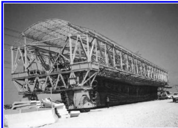
Figure 21. Pre-assembly of reinforcement cage of Padulicella viaduct, Roma-Napoli.
