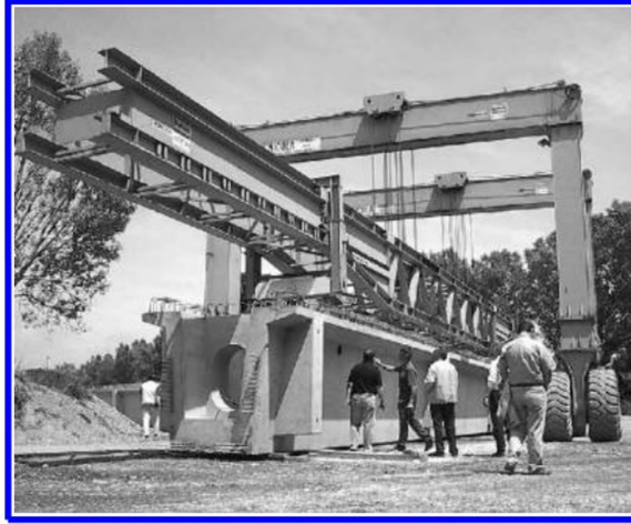
Figure 19. Precast V beam lifted up from stoking area.
