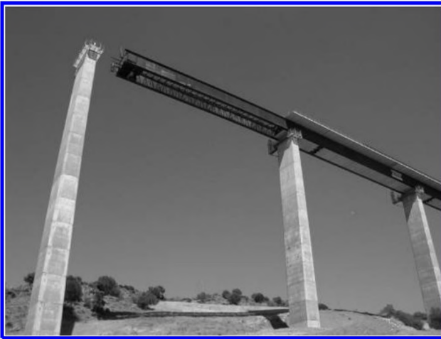
Figure 27. Bridge during launching.
