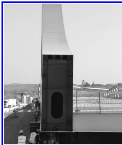
Figure 15. Typical cross-section of the longitudinal beam.
