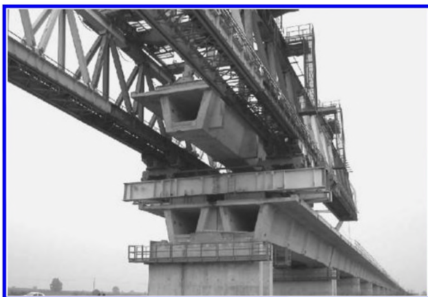
Figure 23. Launching operations of a box girder of S. Rocco al Porto 2 viaduct, on Milano-Bologna line.
