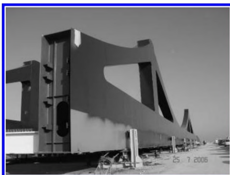
Figure 35. Transverse guides for launching.
