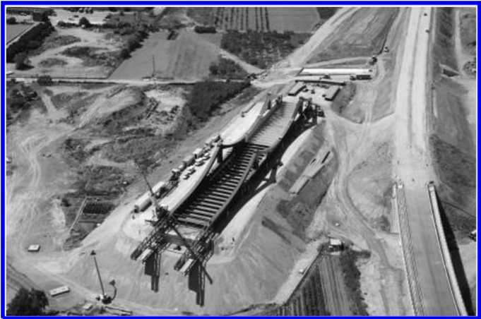
Figure 34. Assembly of the bridge at the site (first segment before launching).
