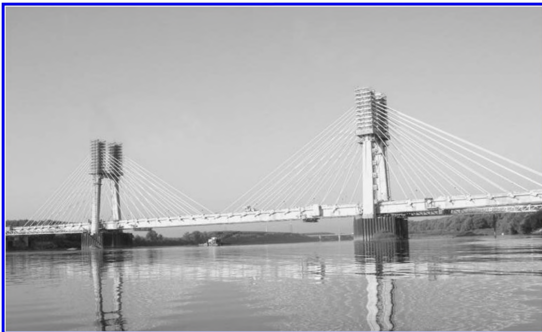
Figure 20. The cable stayed bridge in winter 2006 before removing the cofferdams and the scaffolding at the top of the towers.
