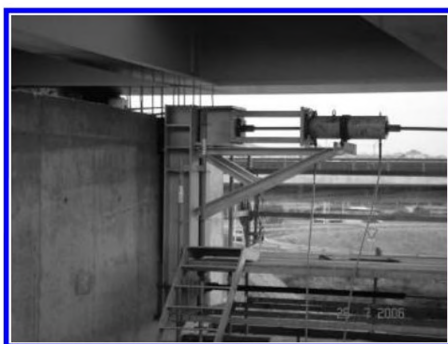
Figure 36. Launching hydraulic jack at abutment.
