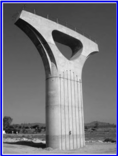
Figure 33. Typical Pier of the concrete viaduct.
