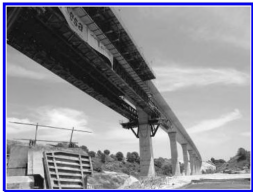
Figure 7. Avernó Bridge. Construction using the span by span method with a total length of 810 m.
