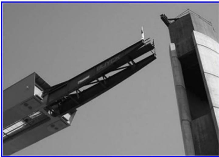
Figure 12. Launching of double box girder of Jaulny Viaduct.
