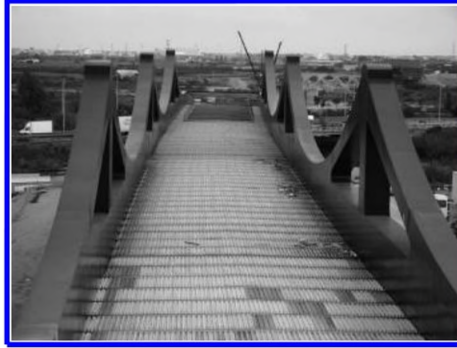
Figure 37. Assembly of the bridge at the site before the second launching phase.
