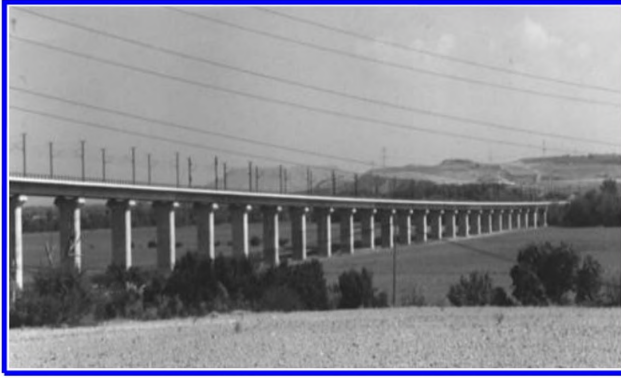
Figure 10. Simply supported precast spans (35 meters long).
