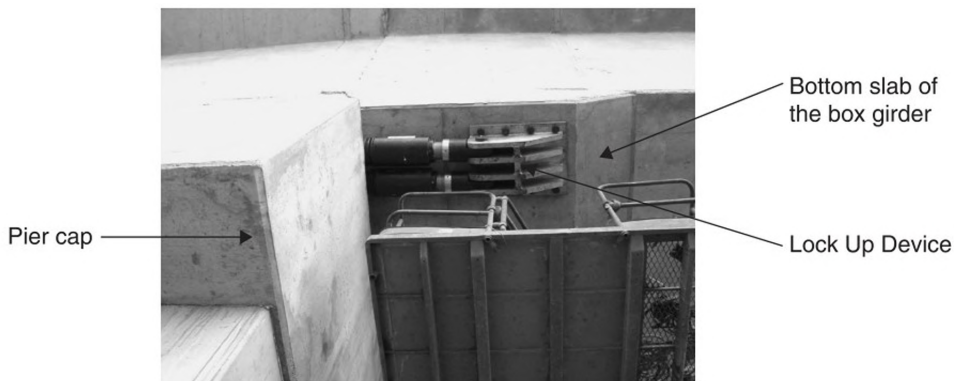
Figure 2. Lock Up Device located between the deck and the pier cap – View from below.
