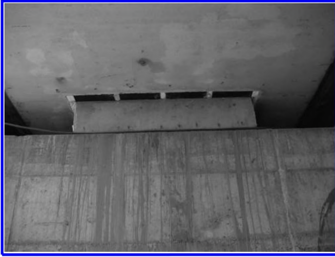
Figure 27. Deck to abutment anchor block.
