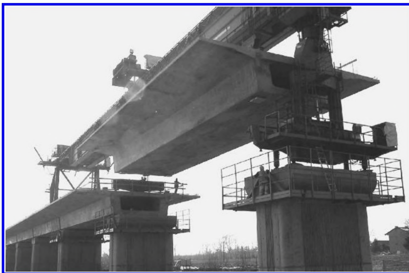
Figure 27. Santhià precast single box deck during launching operations, Torino Milano line.
