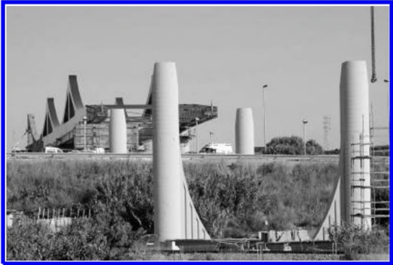
Figure 32. Typical pier of the steel viaduct.
