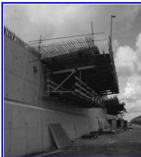
Figure 10. Side view of approach bridge, casting of concrete deck.
