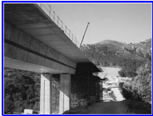
Figure 6. Vandellós Bridge. Construction using the span by span method with a total length of 410 m.
