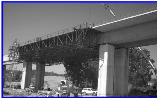
Figure 10. Erection of a beam and typical cross-section of the deck.
