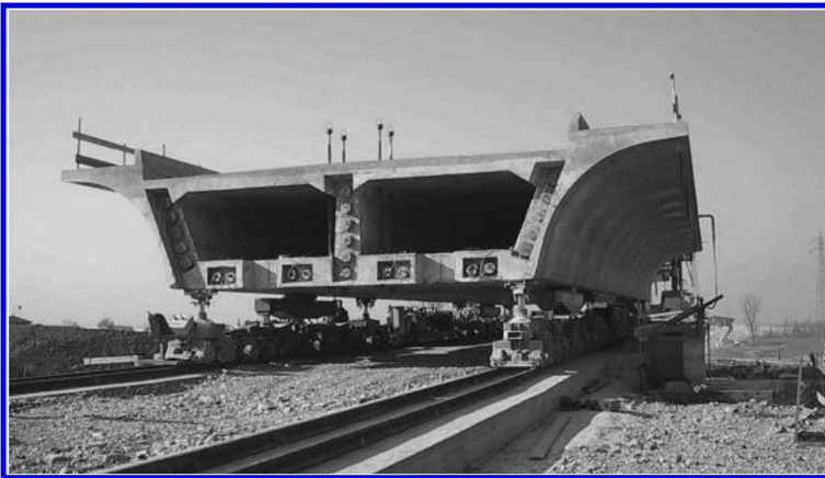
Figure 25. Piacenza precast transported on steel wheels from stocking area towards launching, Milano-Bologna line.
