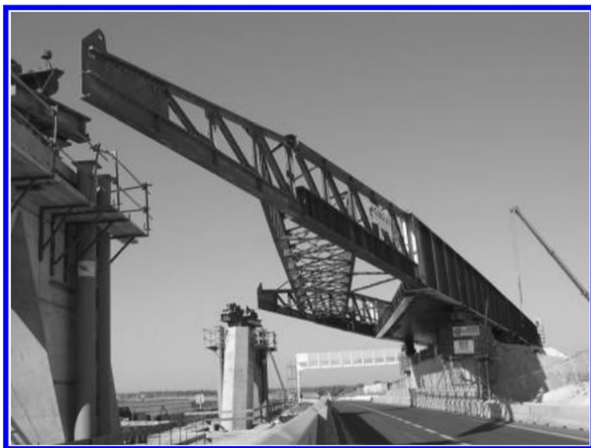
Figure 11. Launching of Orxois bridge over A4.
