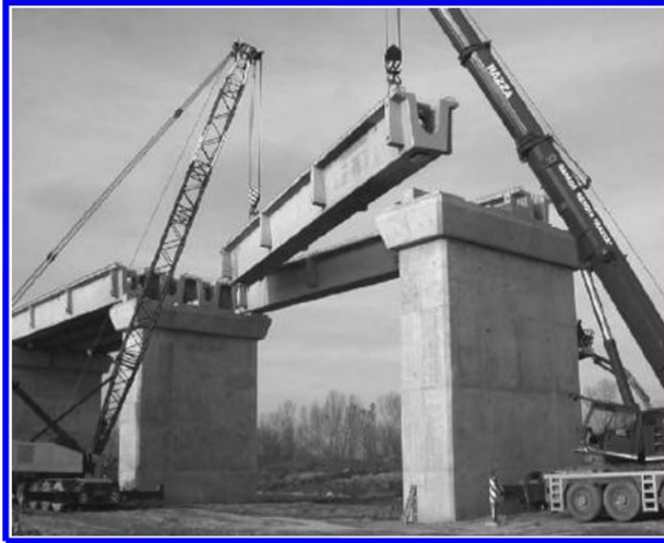
Figure 20. Precast V beam towards final position over the piers.
