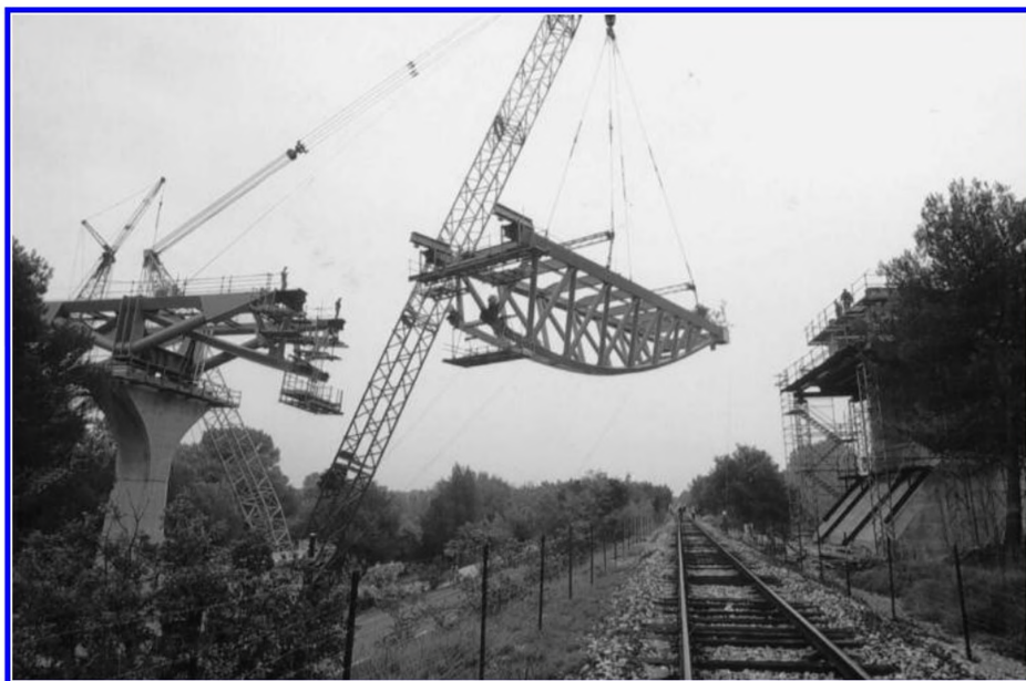
Figure 10. Craning of truss girder bridge.
