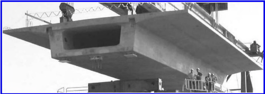
Figure 5. The first precast 25 m long single box girder (Torino – Milano), during launching operations.
