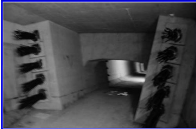
Figure 26. Cables for service conditions anchor blocks in incrementally launched viaduct.
