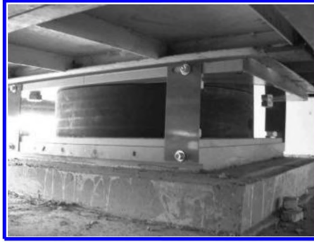
Figure 11. Antivibrating bearing for the Taiwan High Speed Railway.
