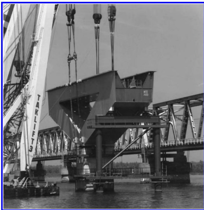
Figure 8. Erection of hammer-section.
