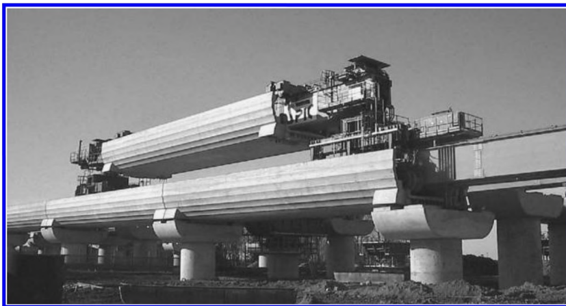
Figure 26. Modena precast lower way U deck during launching operations, on Milano-Bologna line.
