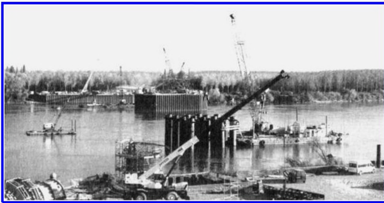
Figure 9. View of the main foundations under construction.
