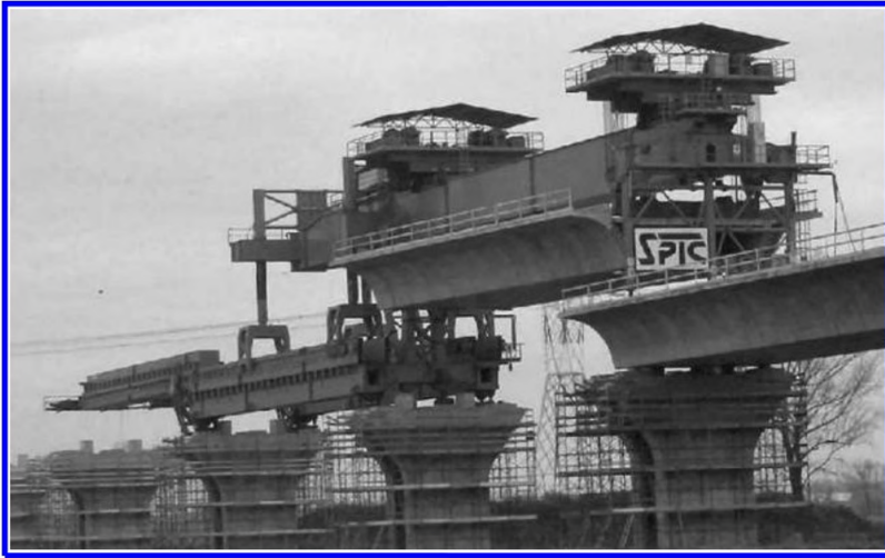
Figure 28. Piacenza precast box girder with two cells during launching operations, on Milano-Bologna line.
