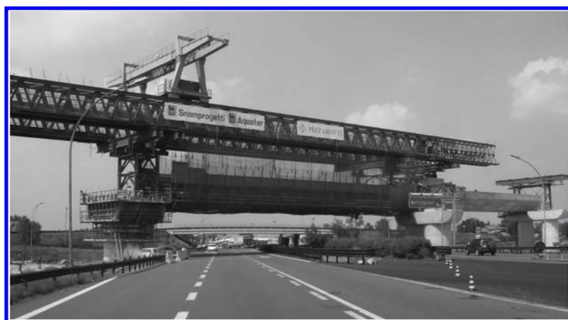
Figure 30. Continuous PC beam of Modena viaduct over Brennero highway, Milano-Bologna line.
